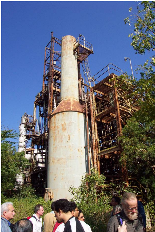
Fig. 10. Photograph of the scrubber system.
