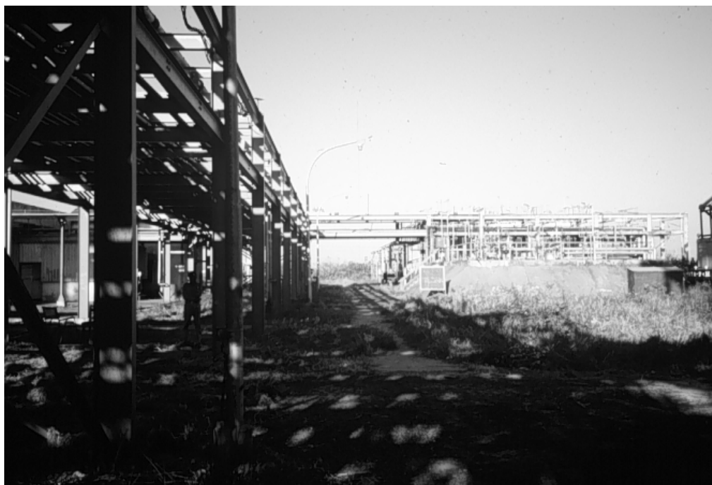
Fig. 3. Photograph taken shortly after the accident. A pipe rack is shown on the left and the partially buried storage tanks (three total) for MIC are located mid photo right.
